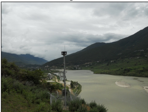
Siren tower above the road between Khuruthang and Wangdue, near Vocational Training Center
